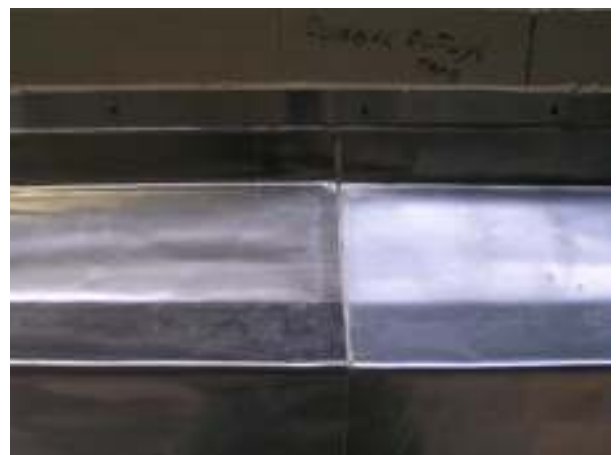
..... or double sided butyl tape. The overlap should be >100mm.
